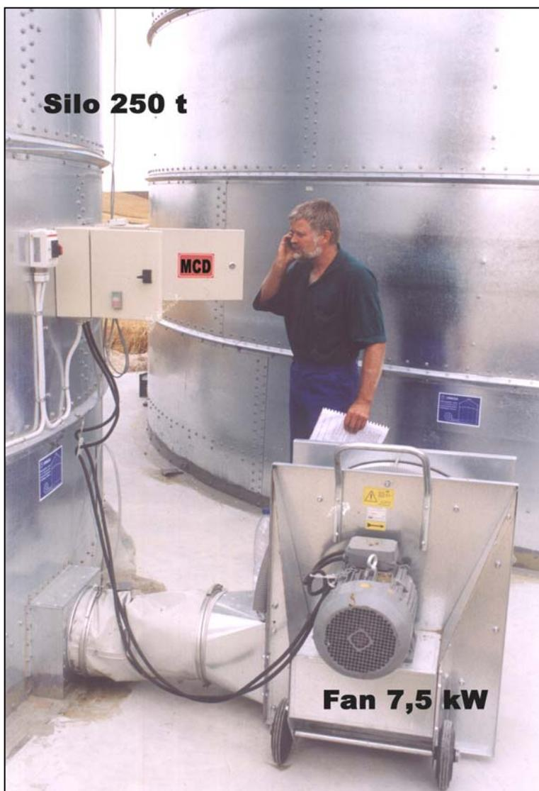
**Figure 3.4. Example of devices** enables the preservation of dry grain with a near-ambient method (courtesy the KBN company, Esbjerg, Denmark).
